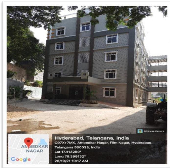
7.1.7.1. Build Environment with Ramps at Hostel -3
