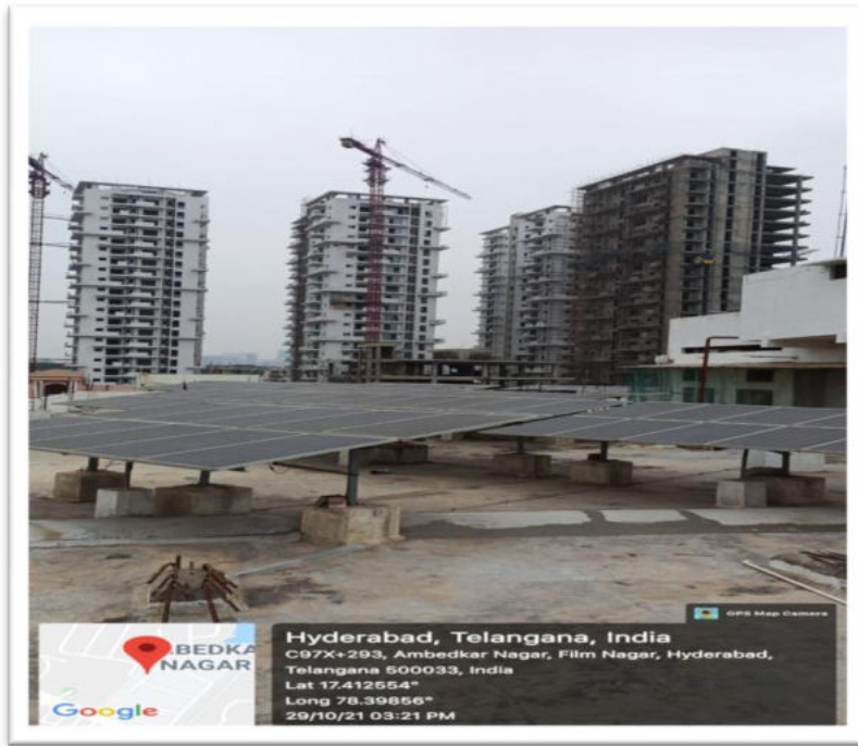
7.1.2.1. Solar Energy – Solar Panels at Admin – Block Terrace
