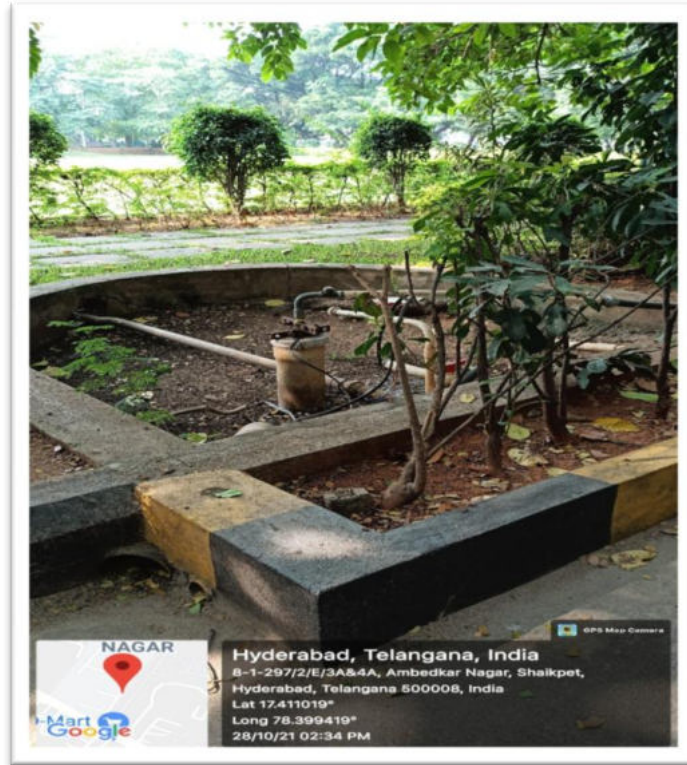
7.1.4.1. Rain Water Harvesting Pit at Busbay
