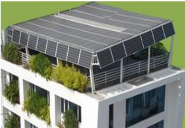
Watts Peak. Solar panels at Synergy Infra, Hyderabad
